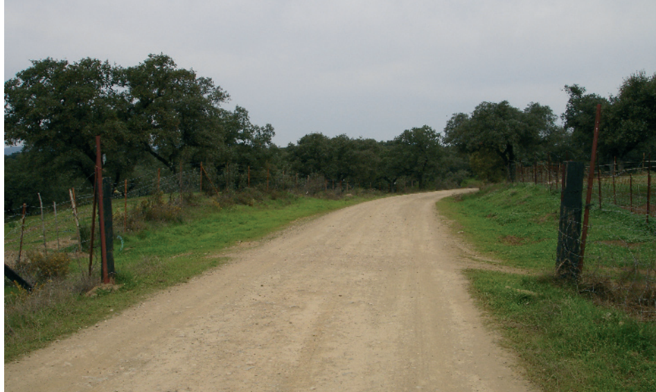
El camino es una pista de zahorra compactada en buen estado. The lane is a track made of compacted graded aggregate material in good condition.
